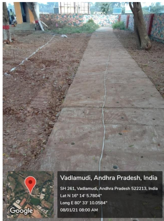
Fig 18. Closed Drain system at VFSTR campus
